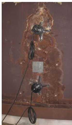
Figure 18 Installation of a Time of Flight (correlation) flow sensor
