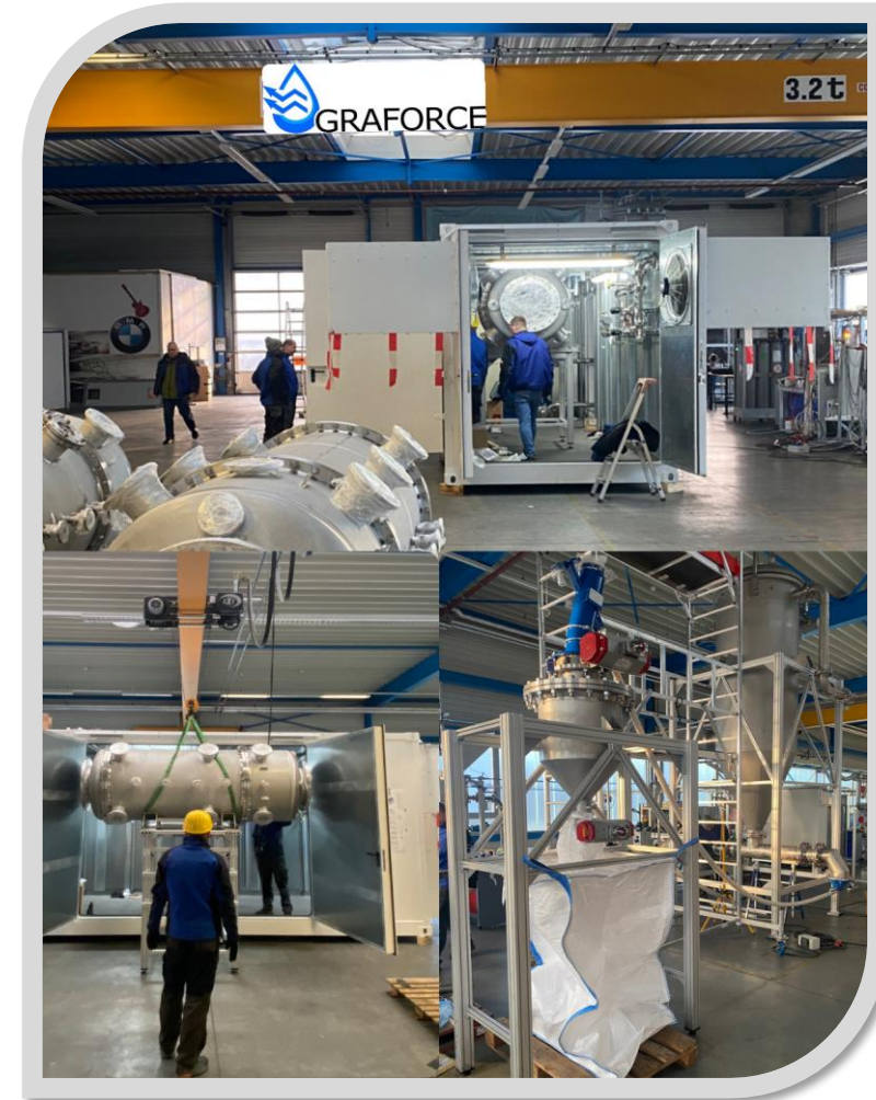
Assembly of a 0.5 MW Methane Plasmalysis plant
